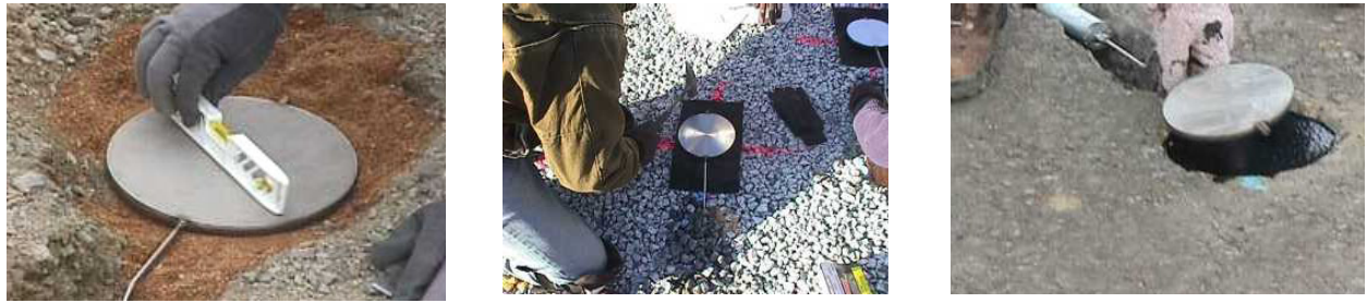
FIGURE 2 Pressure cells installed at different layers within the pavement sections.
